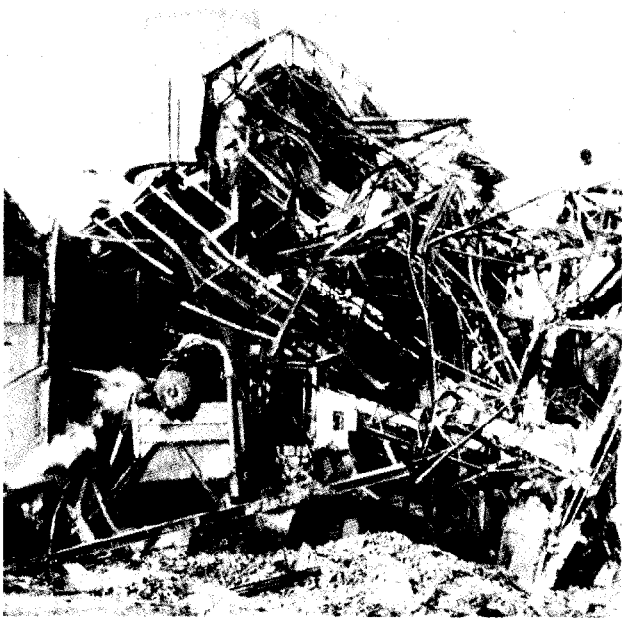
Fig. 1 Power plant after explosion due to caustic embrittlement of steam boiler 26
